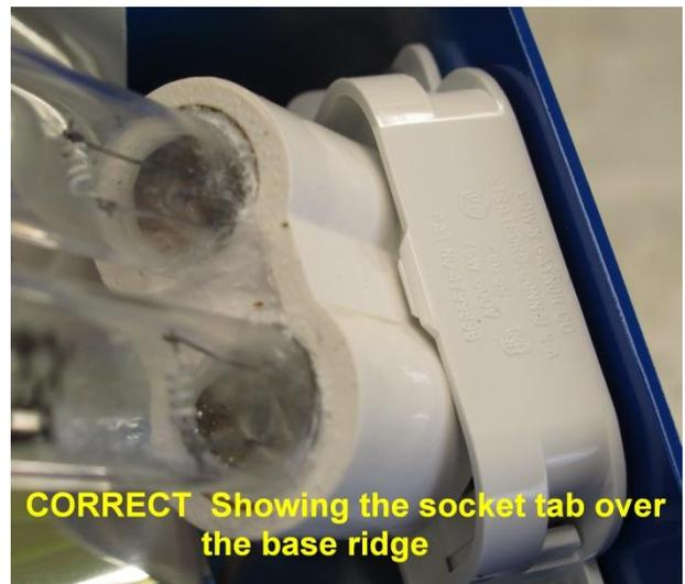
**CORRECT** Showing the socket tab over the base ridge
